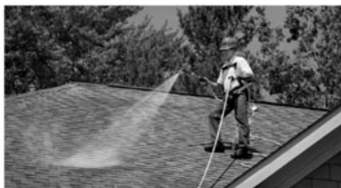
Apply Roof Maxx Protection
