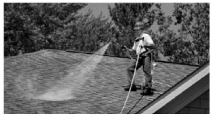
Apply Roof Maxx Protection
