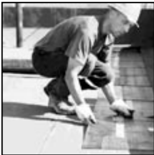
FLAT TOP ROOF
